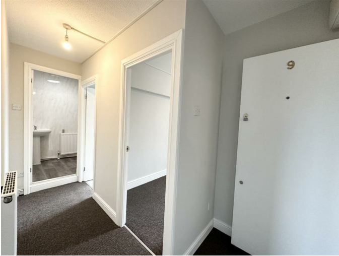
Wooden entrance door & radiator
